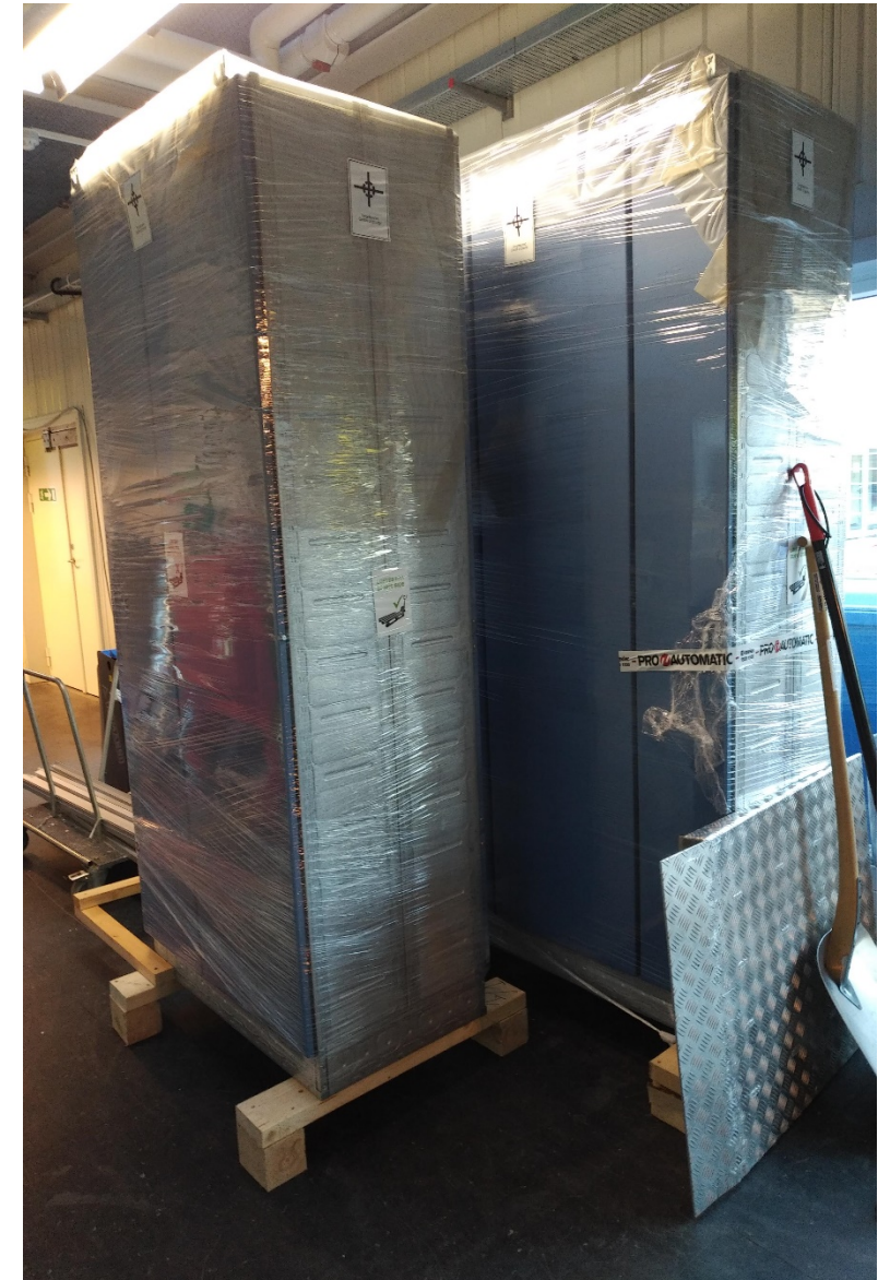
New electrical panels
